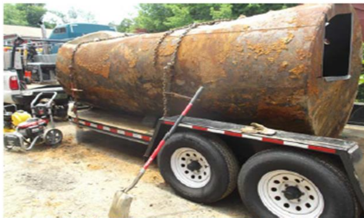
Photo 6 (6-24-13): UST cleaned and staged for offsite disposal.
